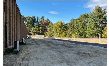
Above: Bus loop road base pavement.
