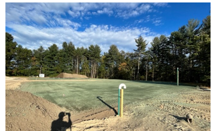
Above: Septic fields loamed and seeded.
