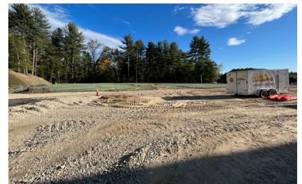
Above: Septic fields loamed and seeded.
