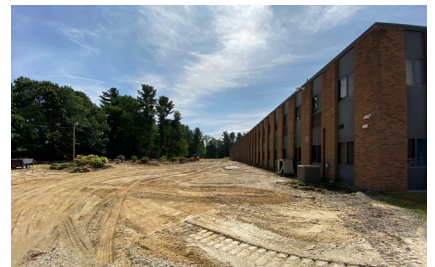
Above: Site work.
