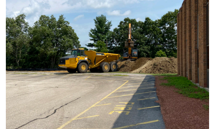
Above: Site work.
